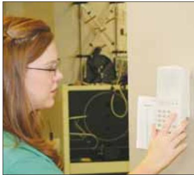
**A staff member at the rehabilitation center demonstrates the facility's new intercom system. Use of the IP intercom products occupy minimal network bandwidth (130kbps maximum) for station-to-station calls and can be controlled and monitored through software or a Web browser.**
