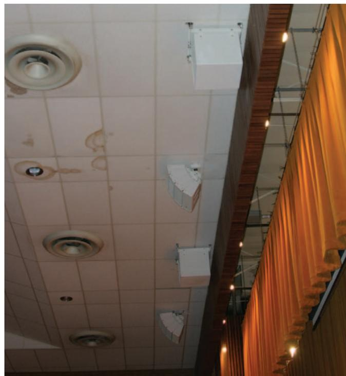
Two TOA FB-120W subwoofers are installed alongside three TOA HX-5W loudspeakers above the theater's curtain line.
